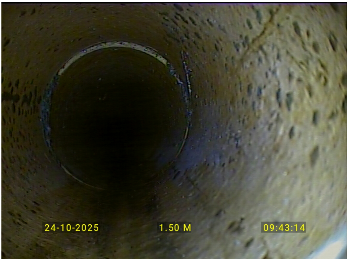
Misaligned pipe on gents basin run
