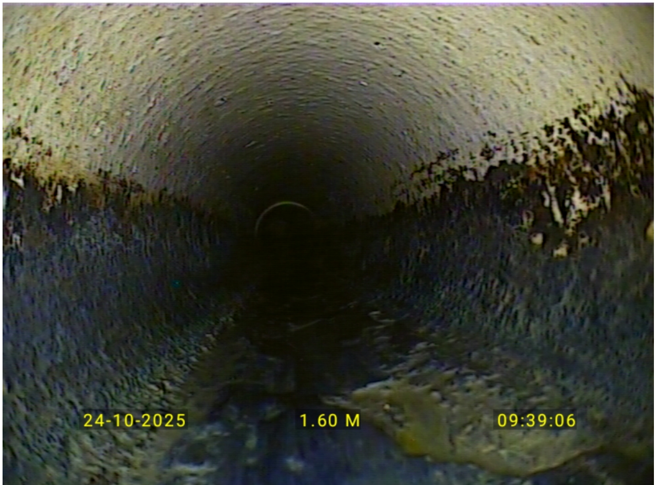
Scale build-up shown in gents toilet run
