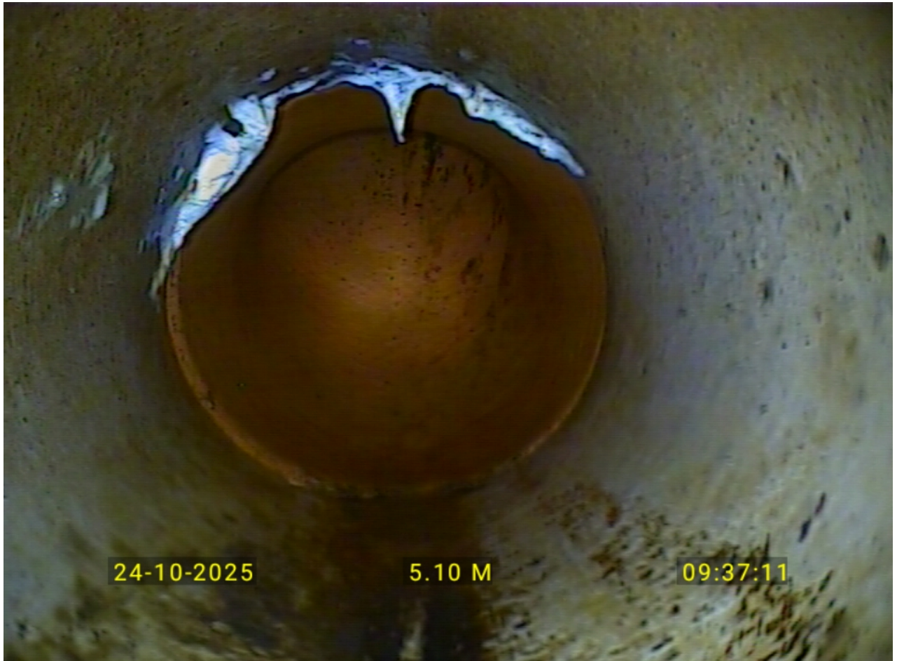
Misaligned joint in gents toilet line
