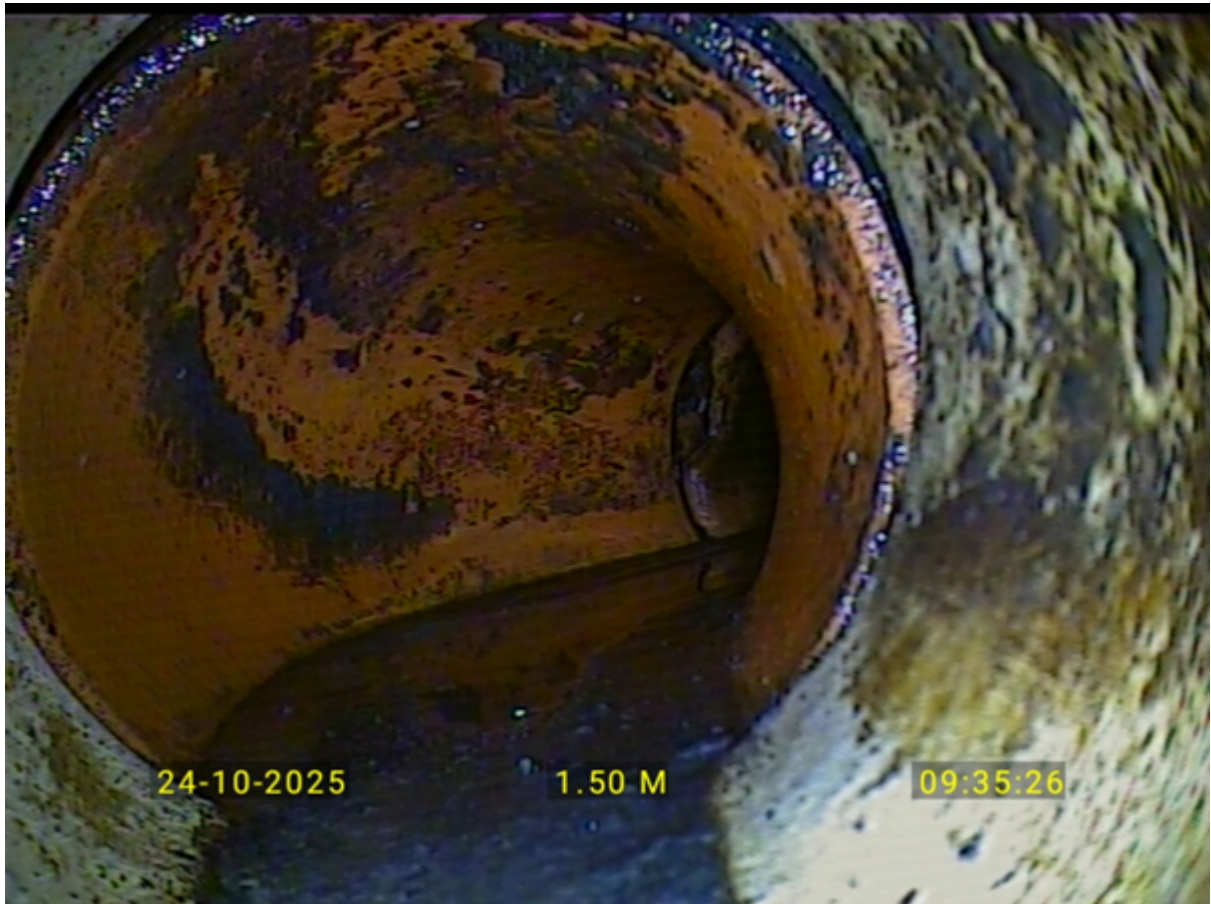
Misaligned pipe with standing water in disabled/ladies
