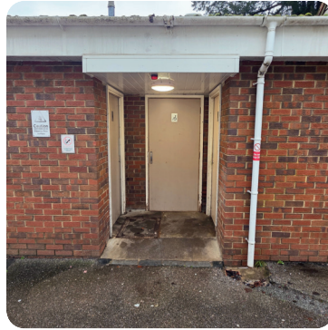
Town centre public toilets
