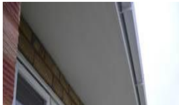
Pieces of Asbestos Insulating Board (AIB)
