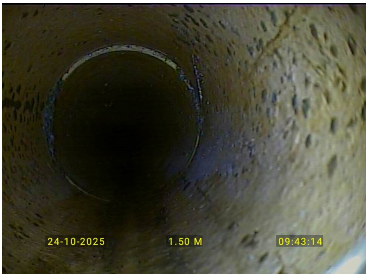
Misaligned pipe on gents basin run
