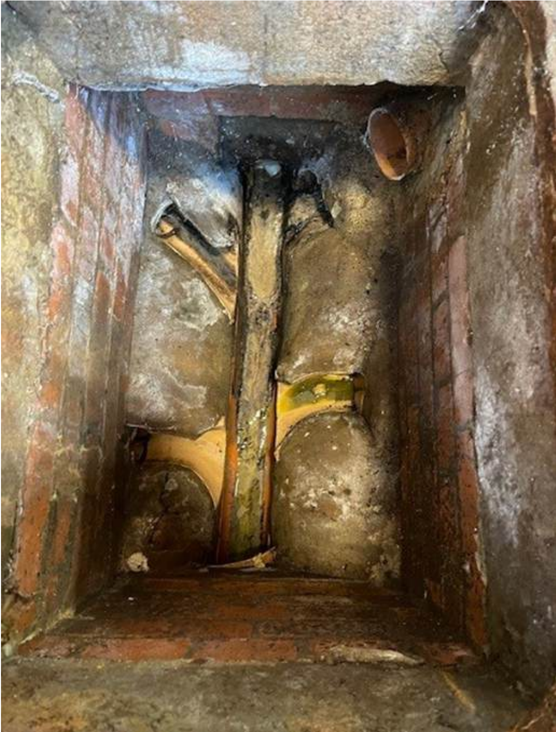
Blockage clear and showing heavy scale
