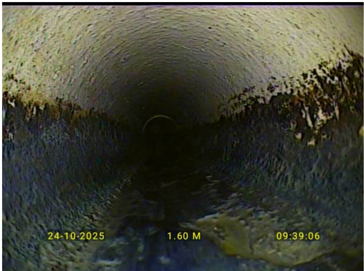
Heavy scale on urinal pipe run
