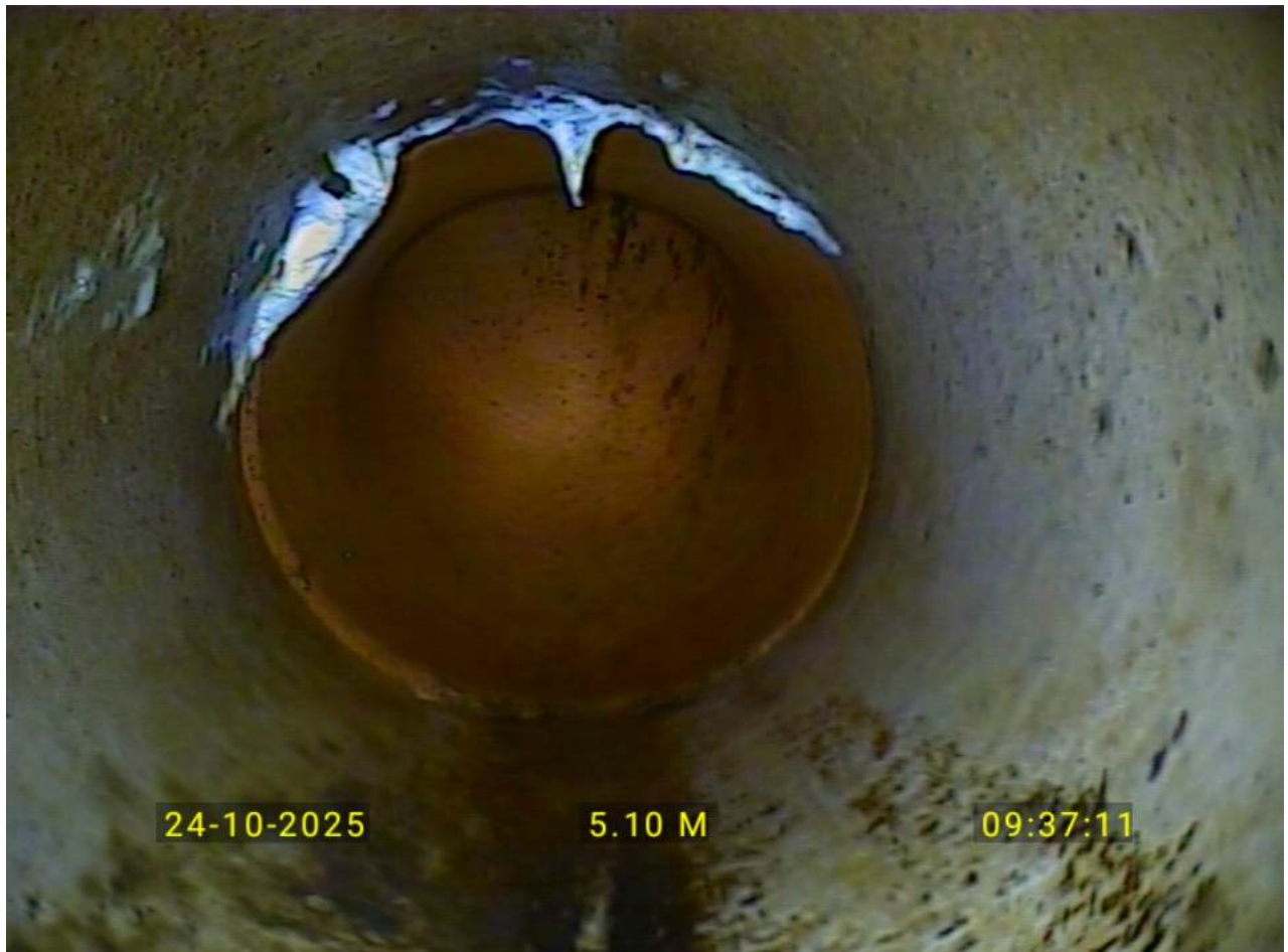
Misaligned joint in gents toilet line
