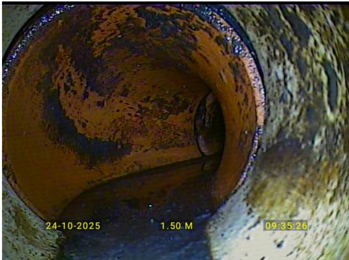
Misaligned pipe with standing water in disabled/ladies
