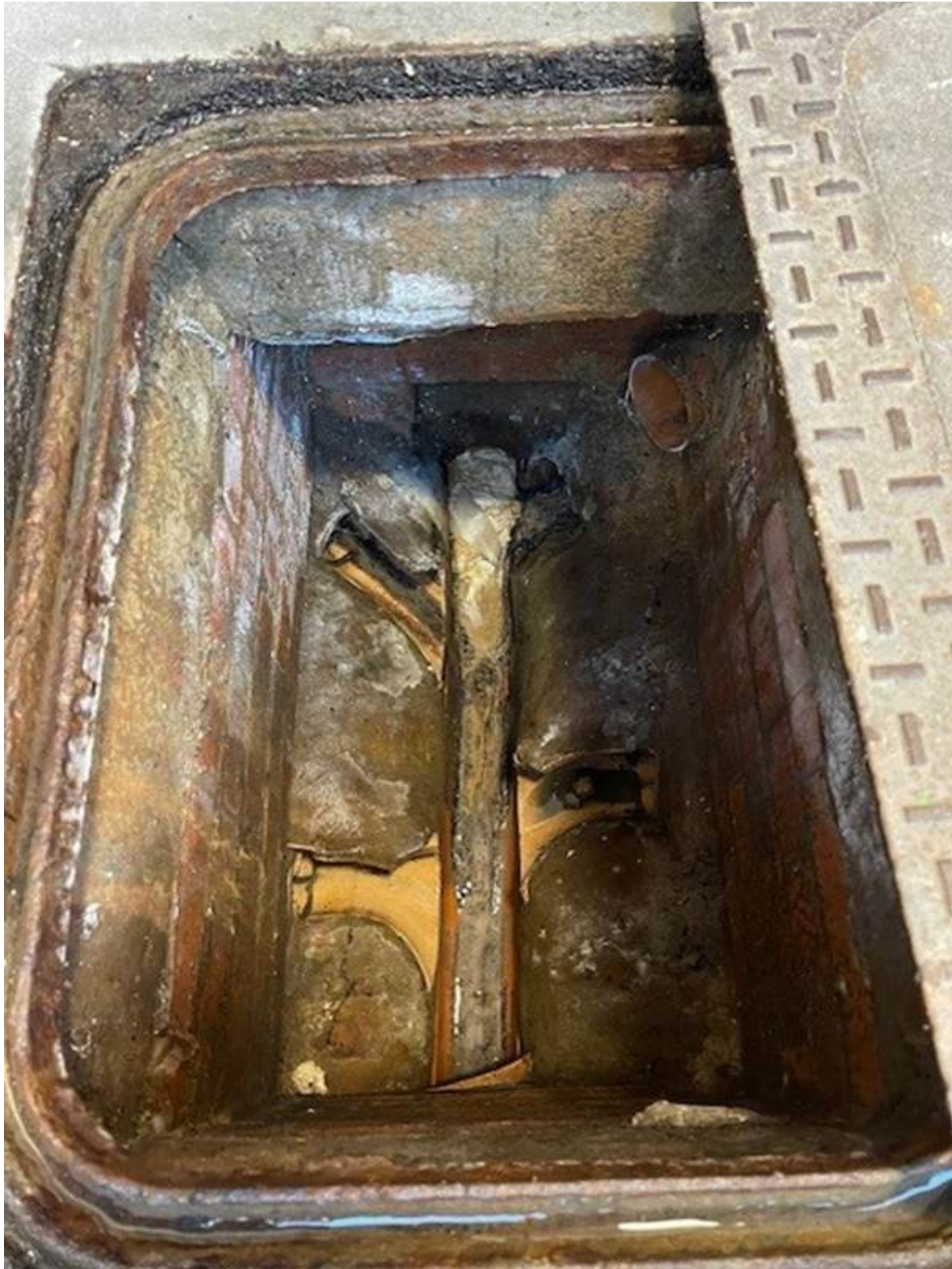
Inspection Chamber with blockages
