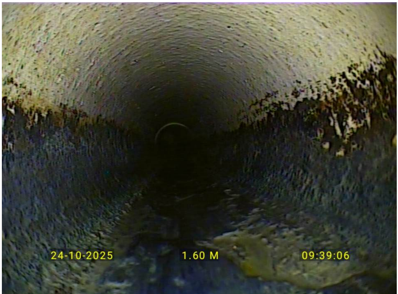
Scale build-up shown in gents toilet run
