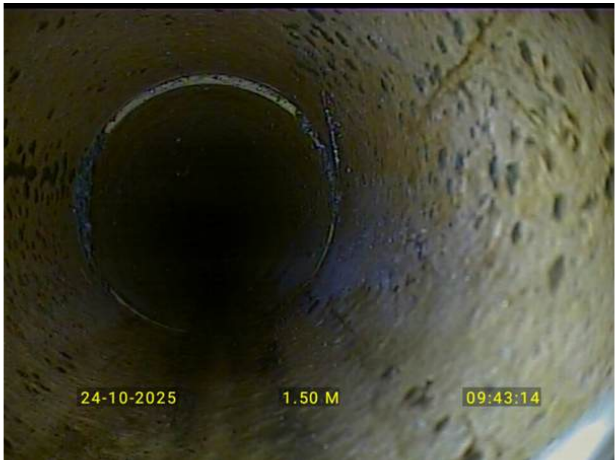
Minor misalignment on gents basin run
